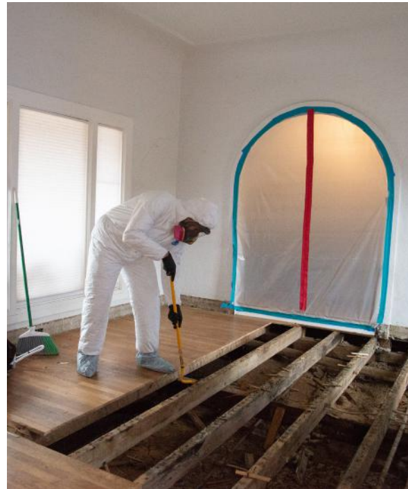
PICTURED: Mold Remediation and Restoration to Family Home
