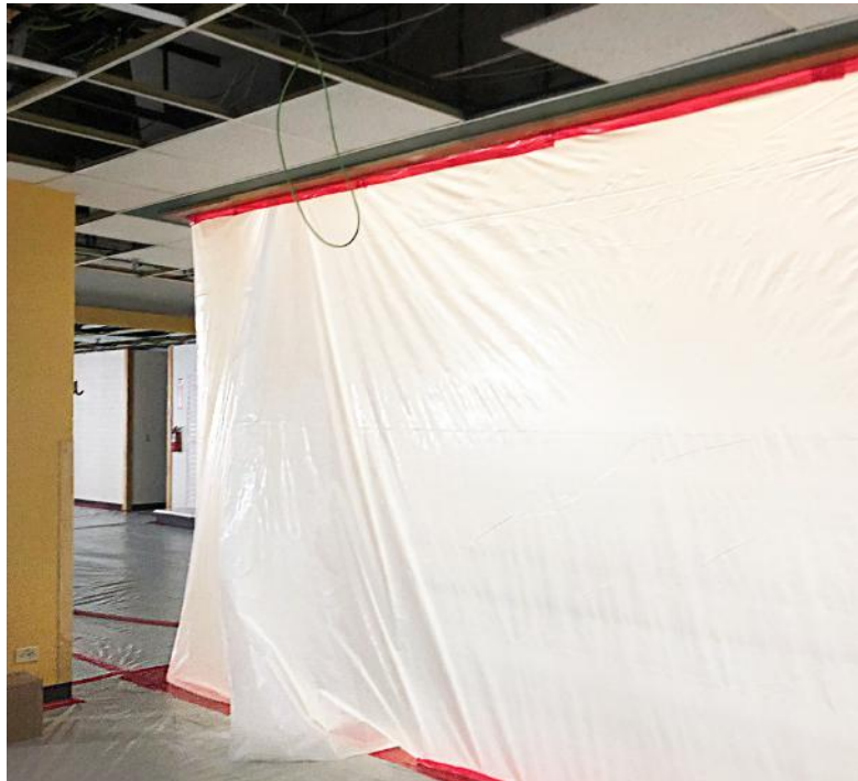
PICTURED: Asbestos Remediation at Colorado State University
