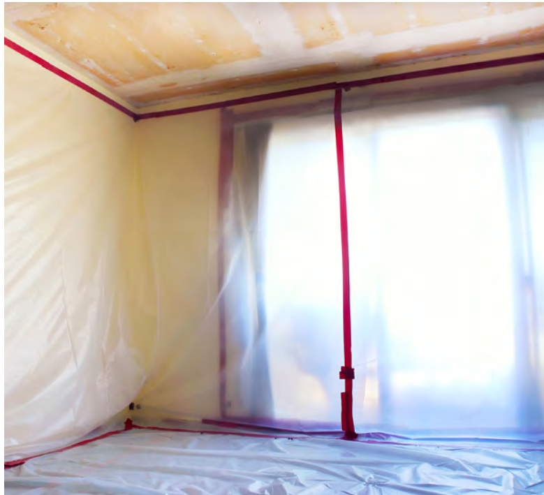
PICTURED: Asbestos Remediation in Family Home
